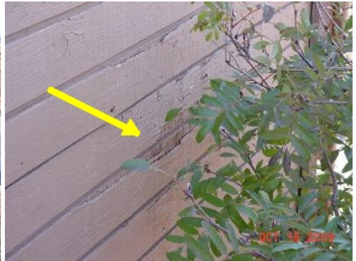
weathered wood siding
