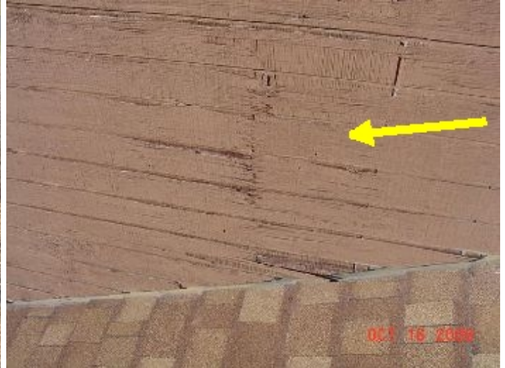
weathered wood siding
