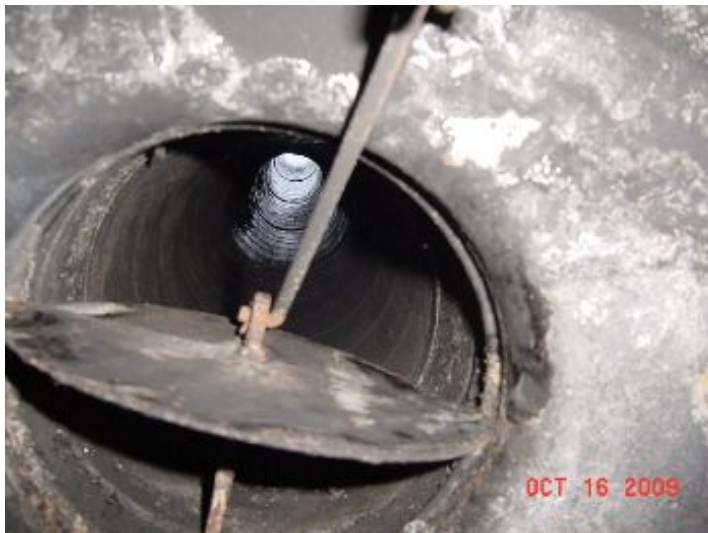
Fire Place Damper & Flue Pipe
