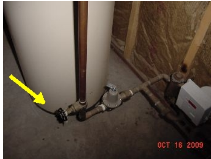
Water Main shut off to house
